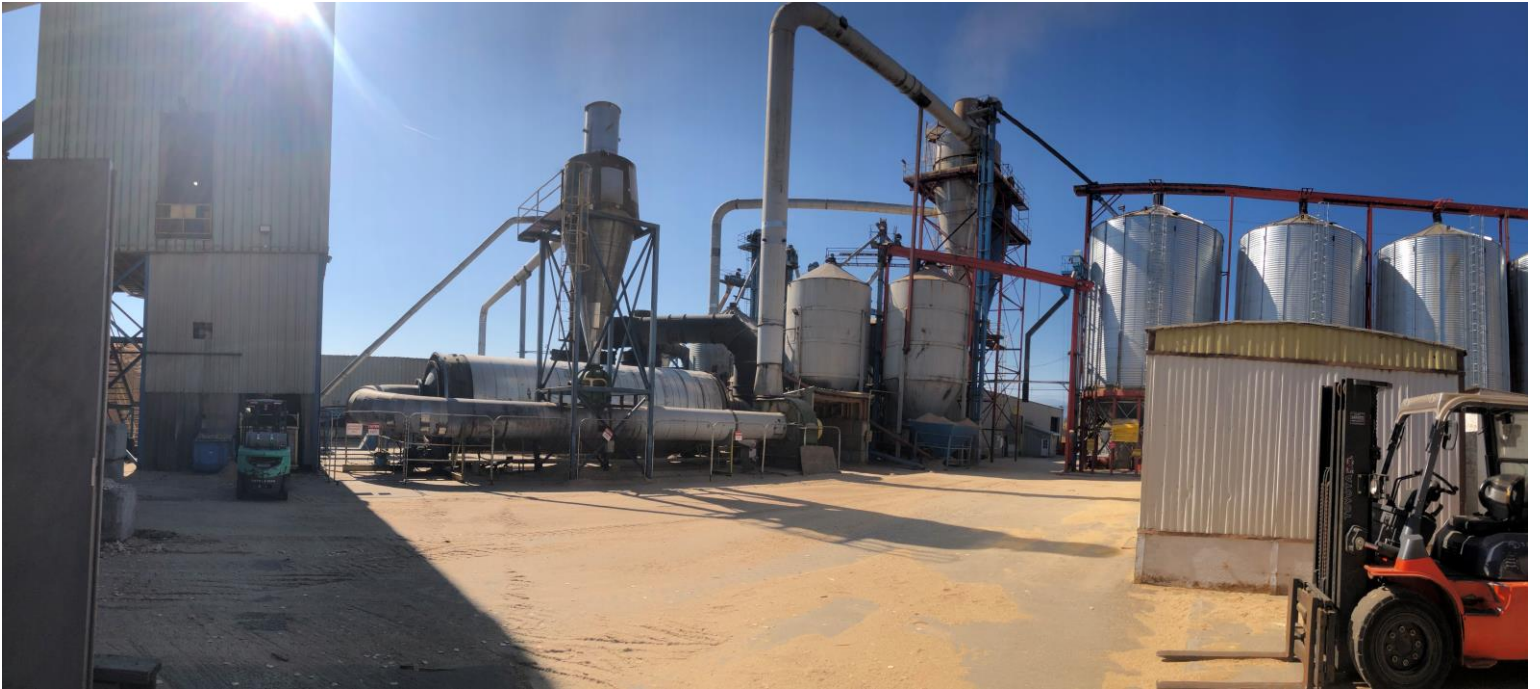
Wet side hammermill tower feeding into dryers and pellet storage silos
