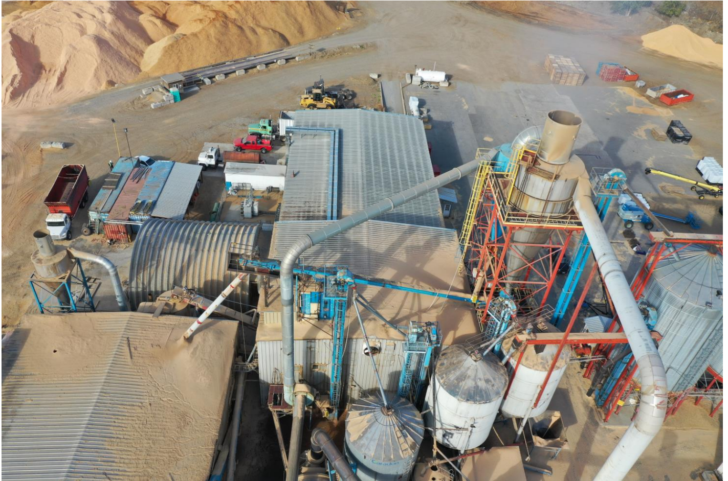
Pellet distribution system using a network of bucket elevators
