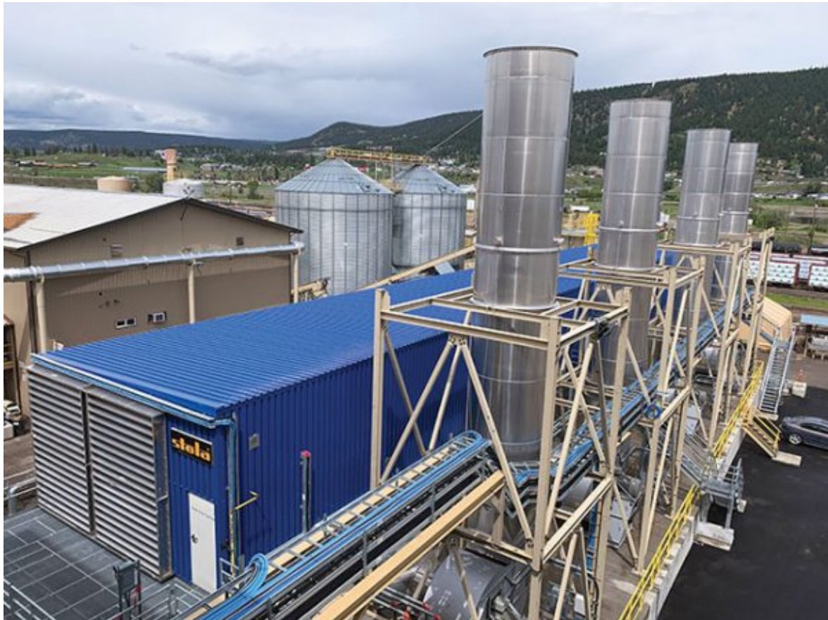
A view of the new Stela bed dryer installed at Pinnacle's Williams Lake plant with the pelleter building and finished pellet storage silos shown in the background.
